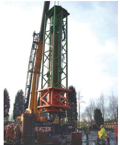
Drill rig prepared for lowering into the ground for testing
