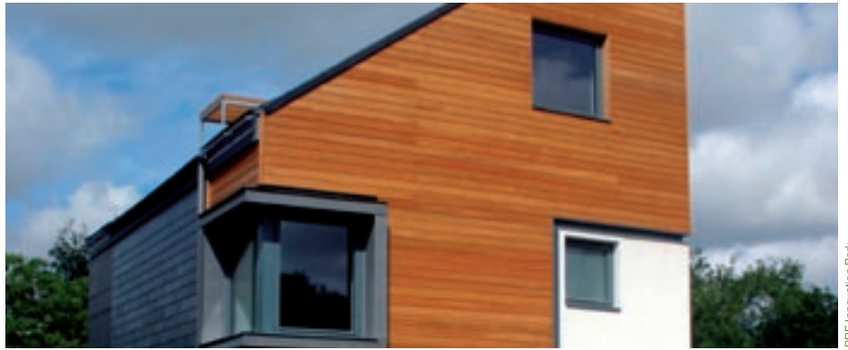
The Code for Sustainable Homes shows how government, taking a long term view, can stimulate innovation, create new markets and deliver policy objectives. This national design and construction standard requires all new homes to be zero carbon by 2016, giving business clarity and an incentive to invest in innovative approaches. Our Low Impact Buildings Innovation Platform is bringing business and government together to focus on this area.
